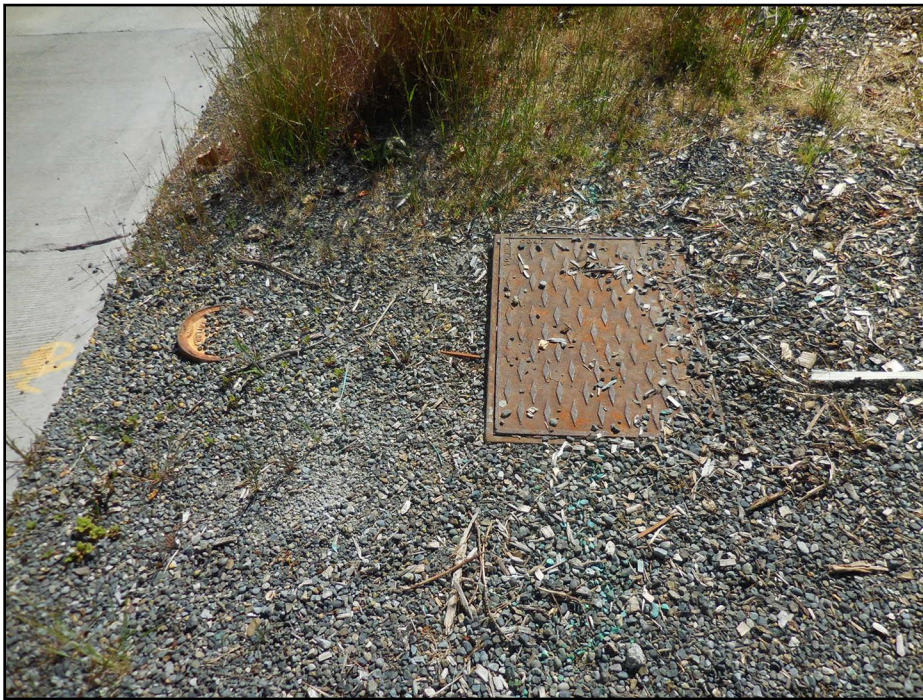
Picture #16: CB 20-61 18" Concrete Pipe IN and 18" CMP OUT
