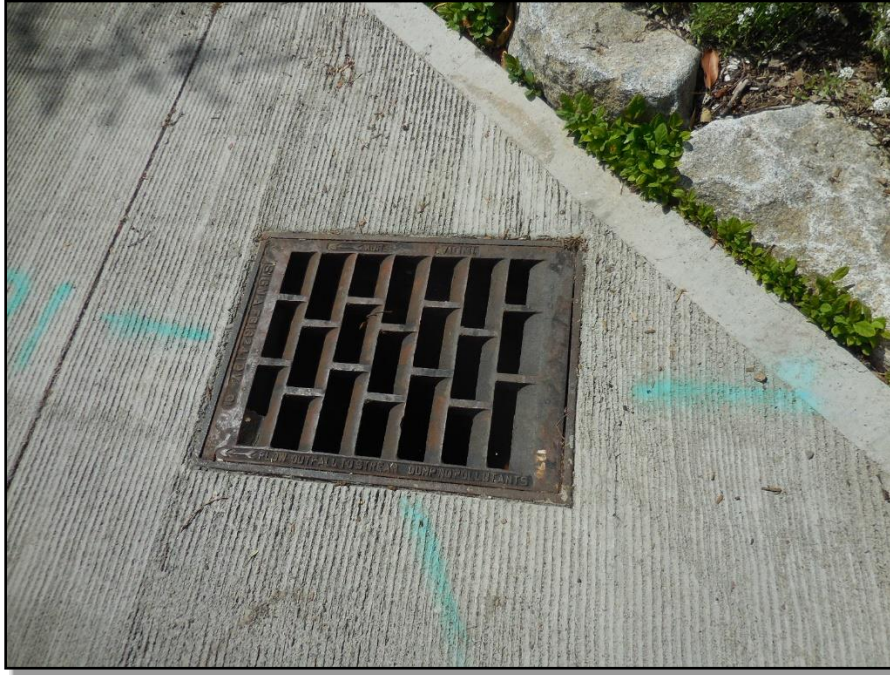
Picture #16: CB 20-61 18" Concrete Pipe IN and 18" CMP OUT
